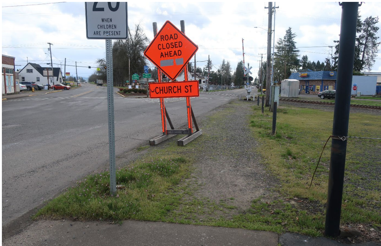
Figure 3. Missing Sidewalk North of the Tricky Triangle
