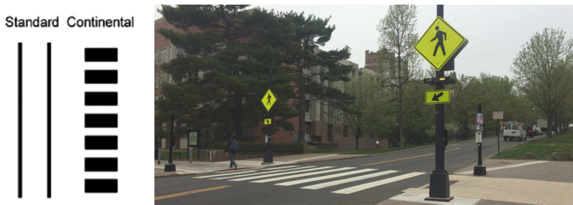
Figure 10. Enhanced Crosswalk Improvements
