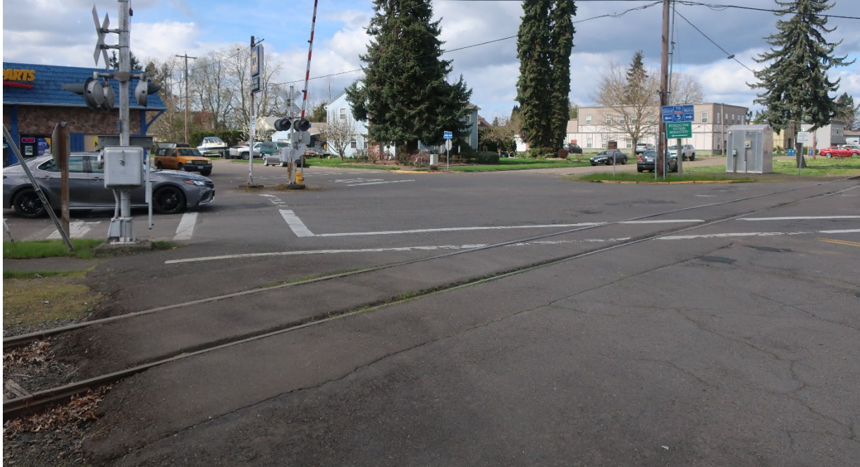
Figure 4. Railroad Crossing at E Church St Adjacent to OR 214 - Uneven Surface, Lacking Sidewalks
